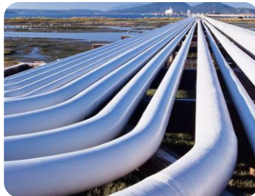
CROSS COUNTRY PIPELINE
